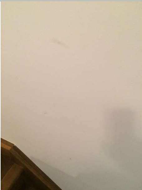
Ground to first floor stair wall
