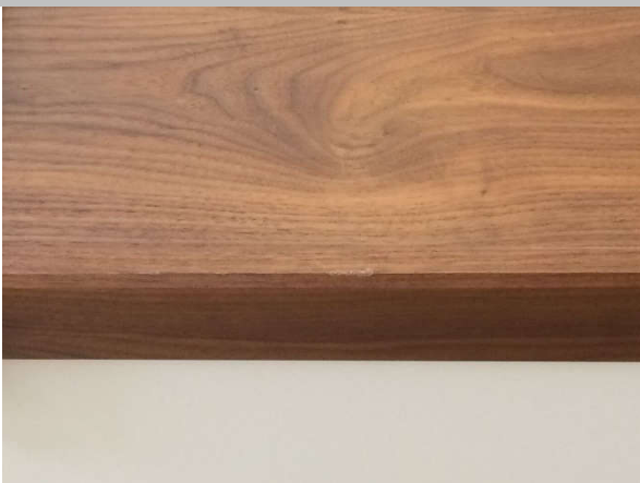
Nosing first floor landing
