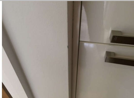
Utility Room wall
