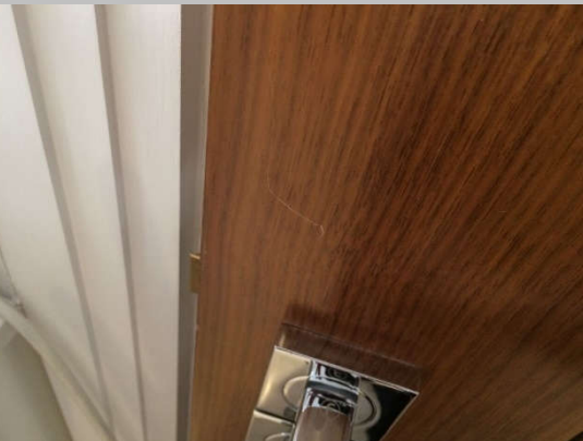
Utility Room Garage door
