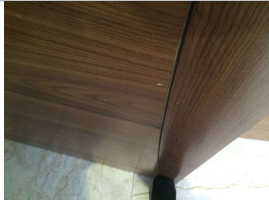
Utility Room Cloakroom door
