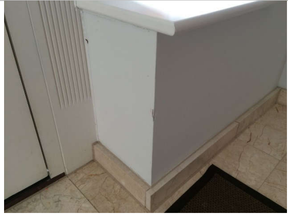
Entrance hall window bay
